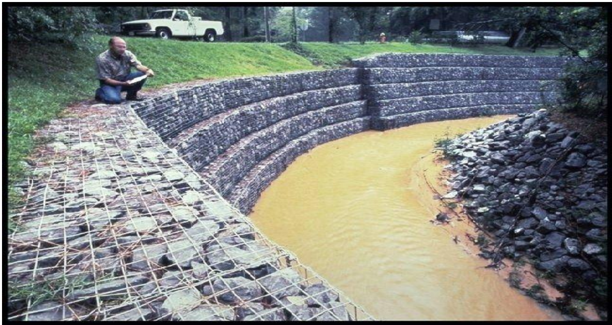
Fig 15: Stream Bank Erosion control by gabion structure
