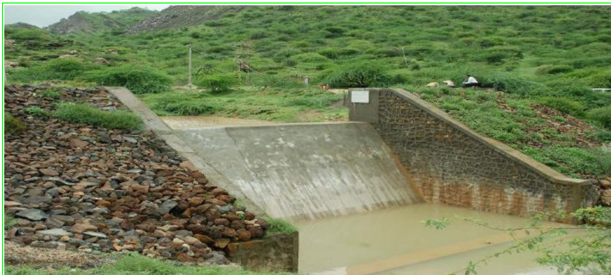
Fig. 51: Masonry Check dam in drainage line
