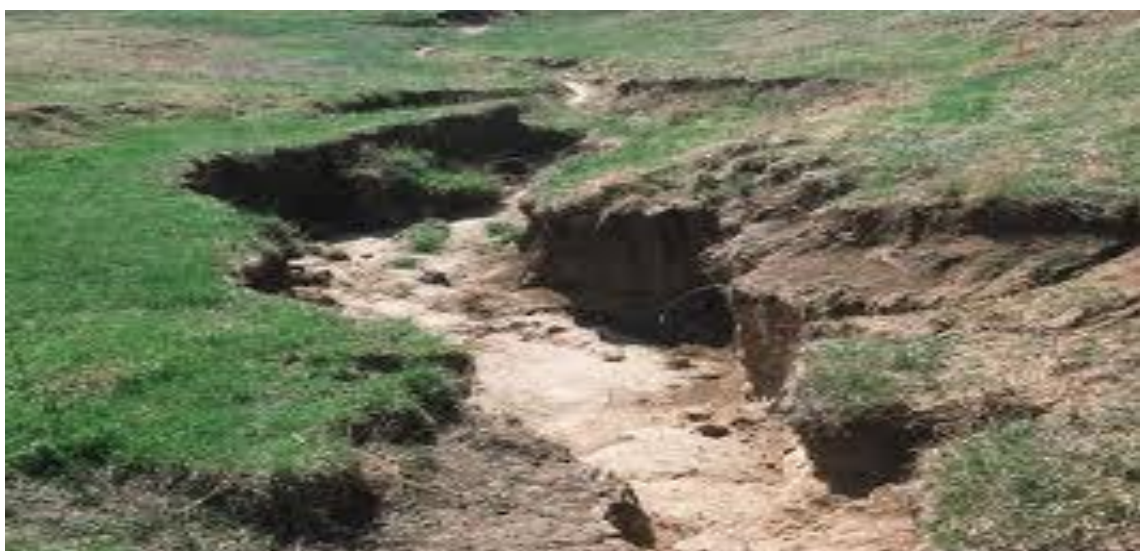
Fig 14: Gully Erosion in the field.
